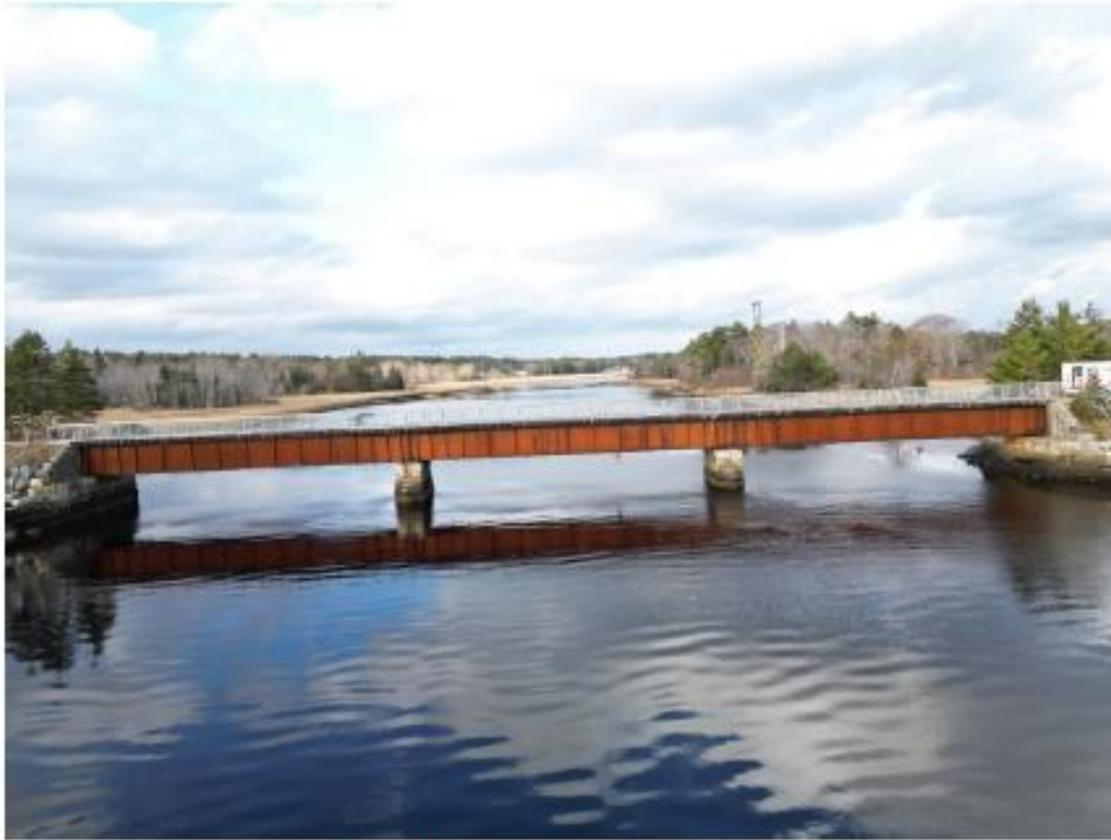
Photo 1: General view – south face.
