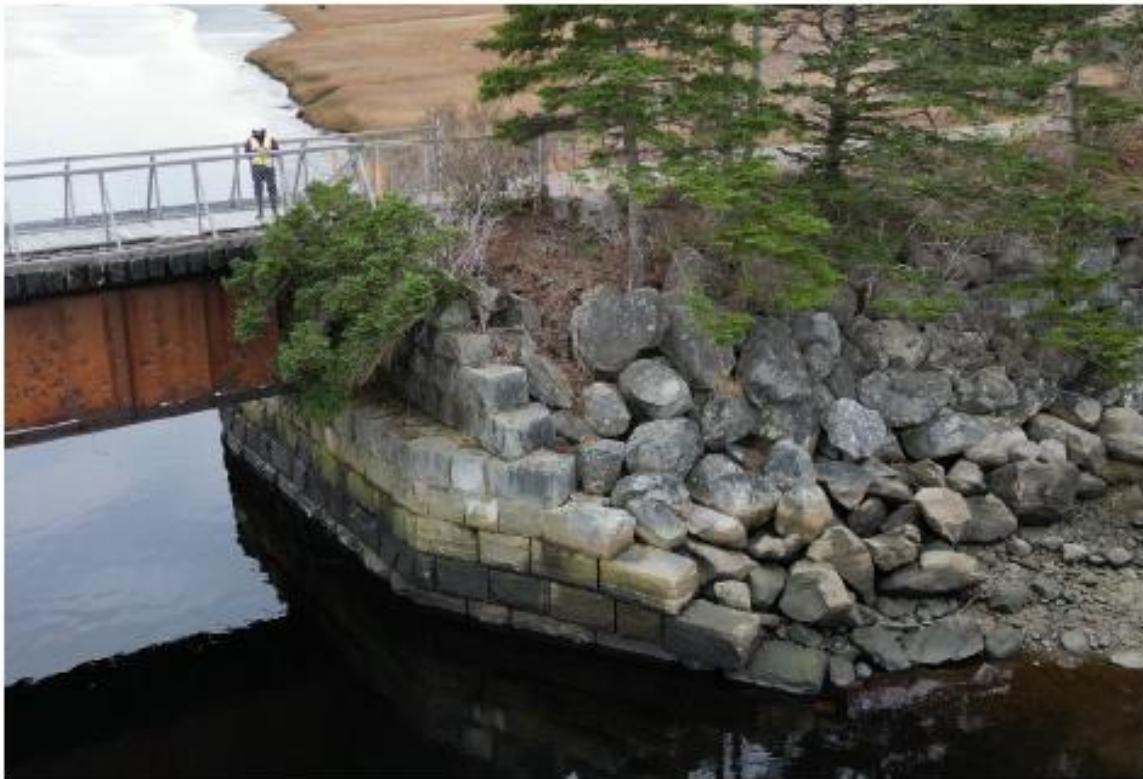
Photo 7: West abutment, north side.
