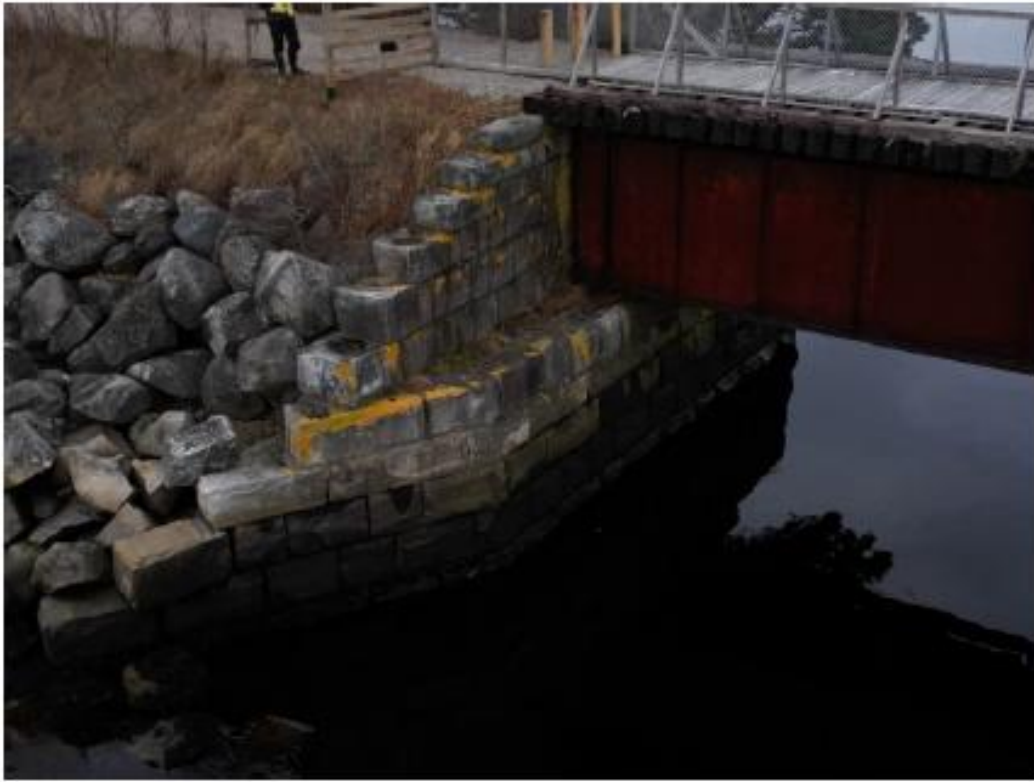
Photo 6: West abutment, south side.
