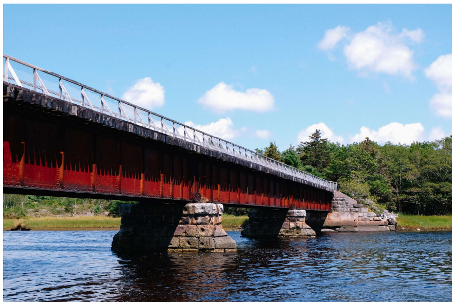
Jordan River Bridge
