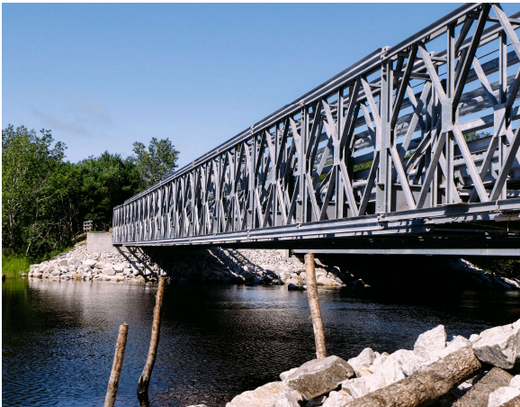
Roseway River Bailey Bridge
