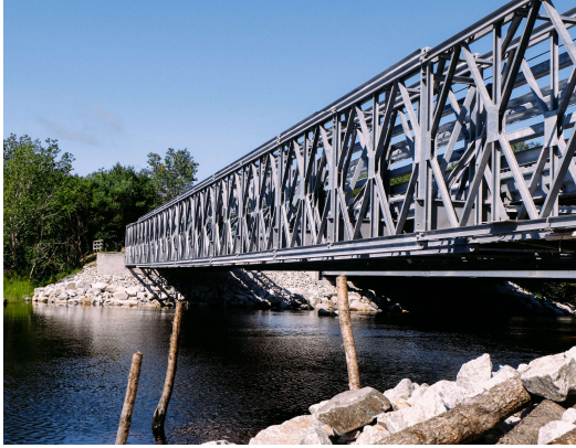
Roseway River Bailey Bridge
