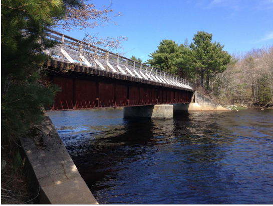
Tom Tigney Bridge
