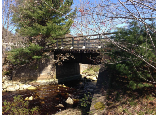
Roseway River Trail Bridge
