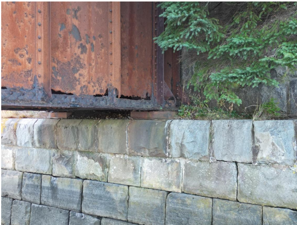
Photo 16: Typical view of superstructure bearings at the west abutment.
