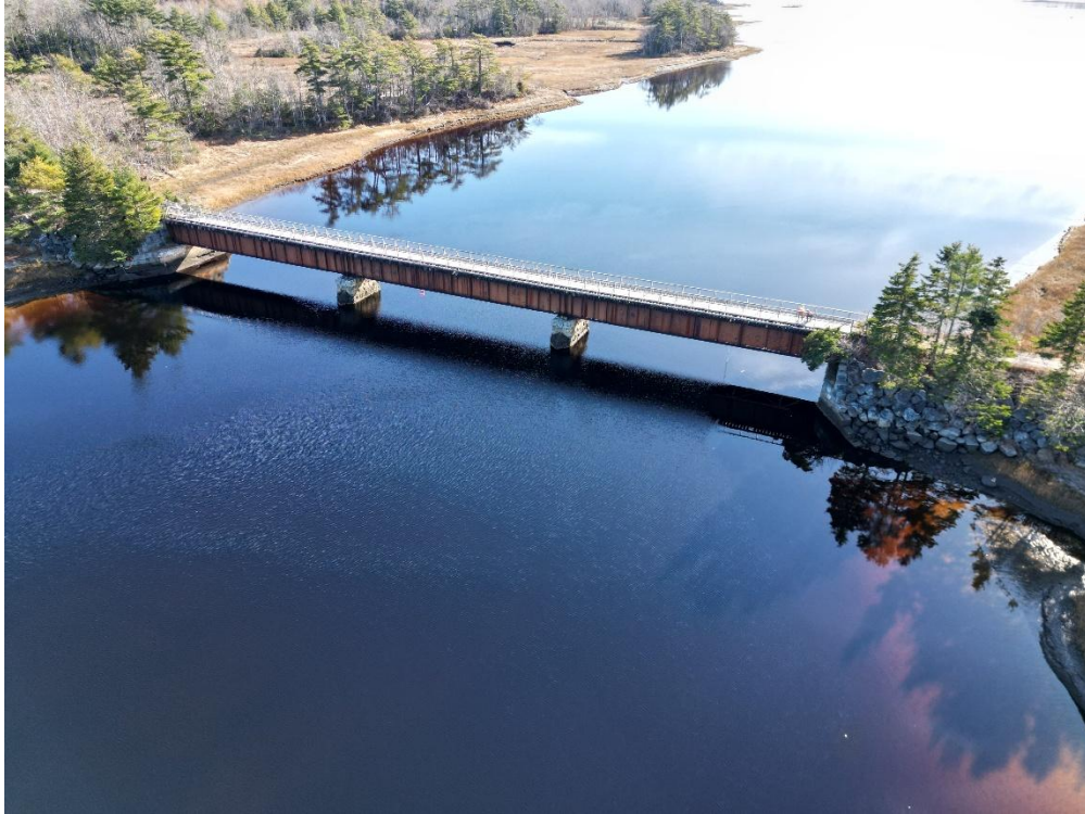
Photo 1: Aerial overview of Jordan River Trail Bridge, facing south.
