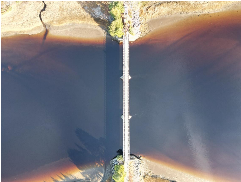
Photo 2: Aerial plan view of the Jordan River Trail Bridge.
