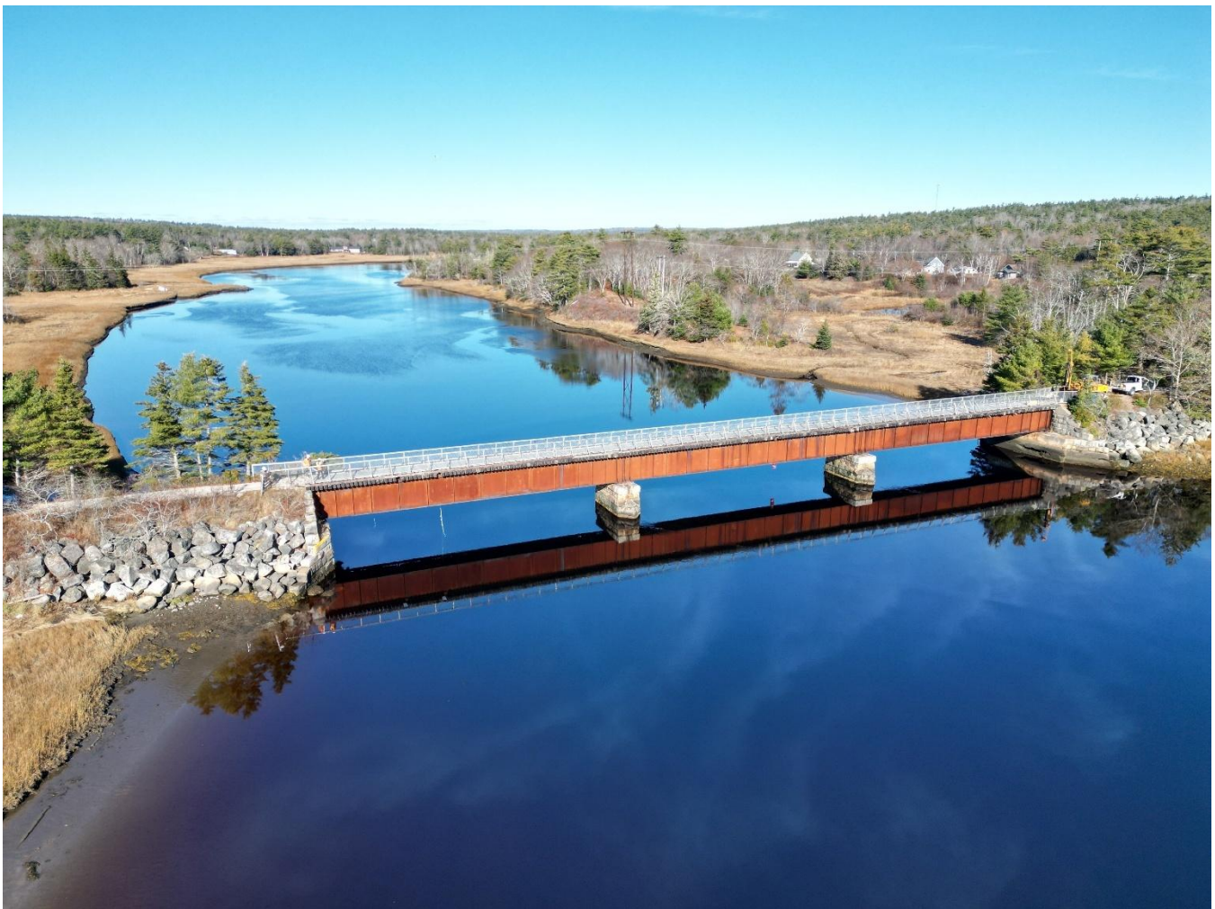
Figure 2 - Aerial view of Jordan River Trail Bridge. Picture facing north.
