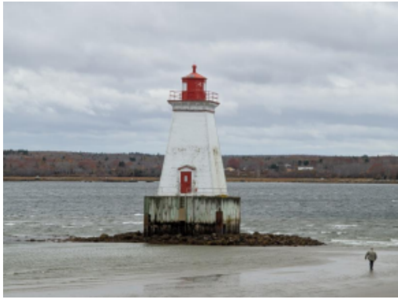
Figure 1: View of the lighthouse from the Sandy Point Recreation Center during low tide
