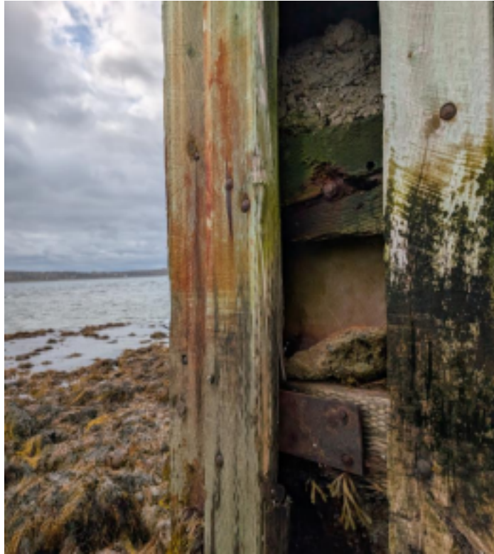
Figure 2: View of the deteriorating and lost timber fenders with the concrete wall behind.
