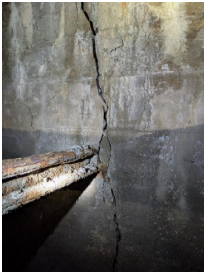
Figure 3: View of typical corrosion of steel bracing and large cracks in foundation wall.
