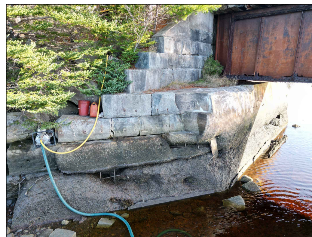
EAST ABUTMENT (NORTH SIDE)
