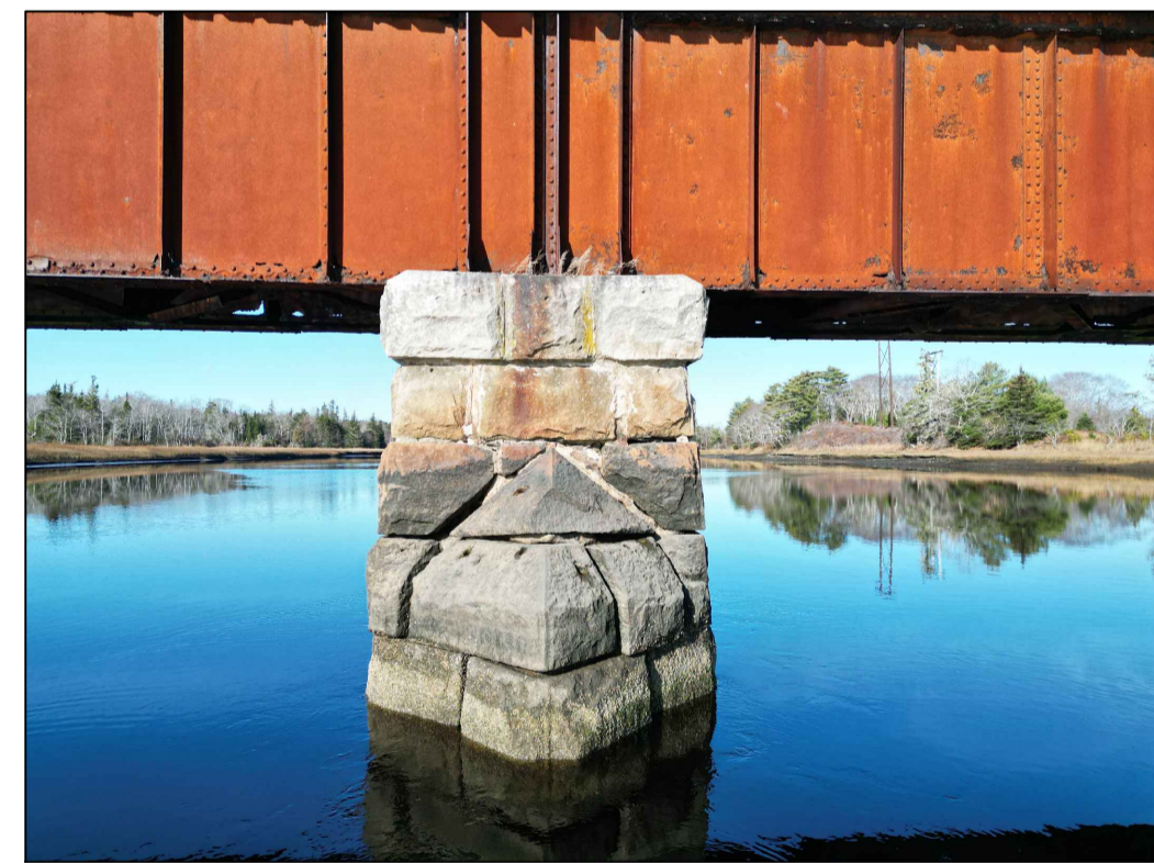
WEST PIER (NOSING)
