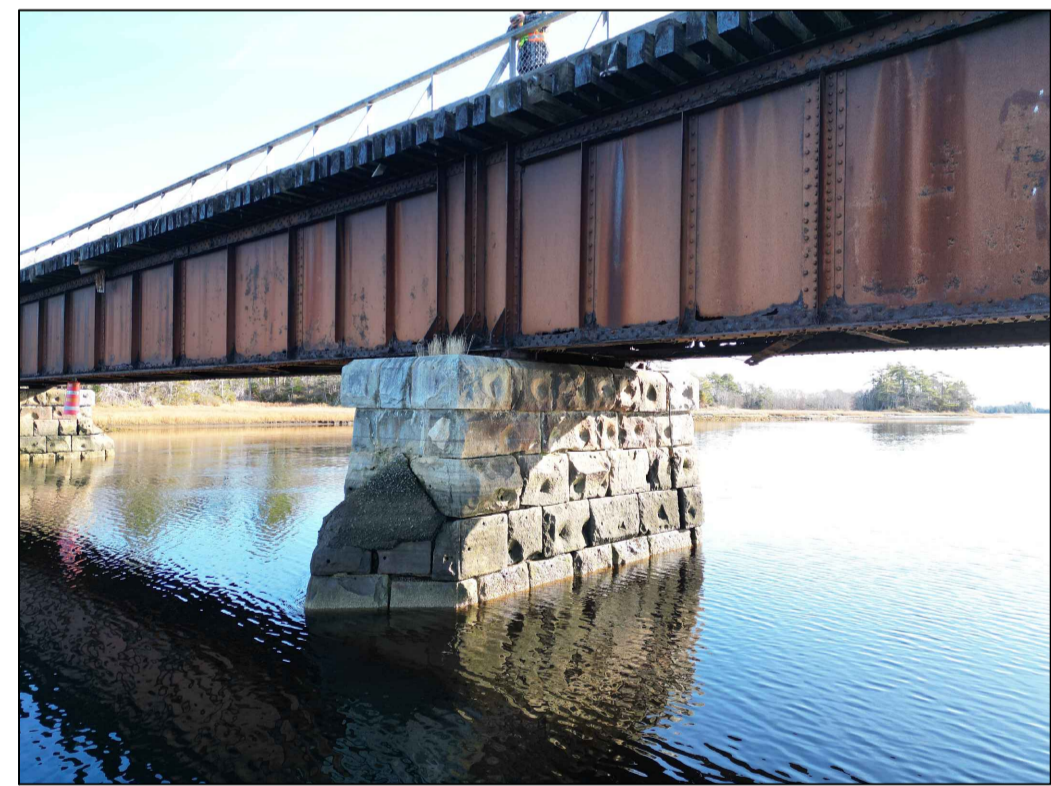
WEST PIER (OVERALL)
