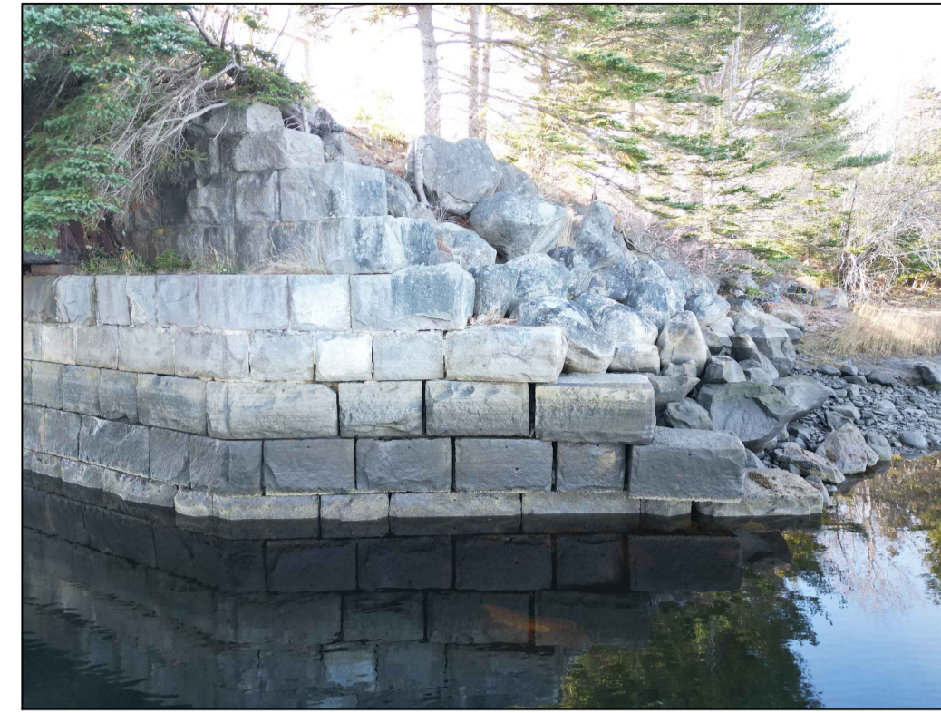
WEST ABUTMENT (NORTH SIDE)
