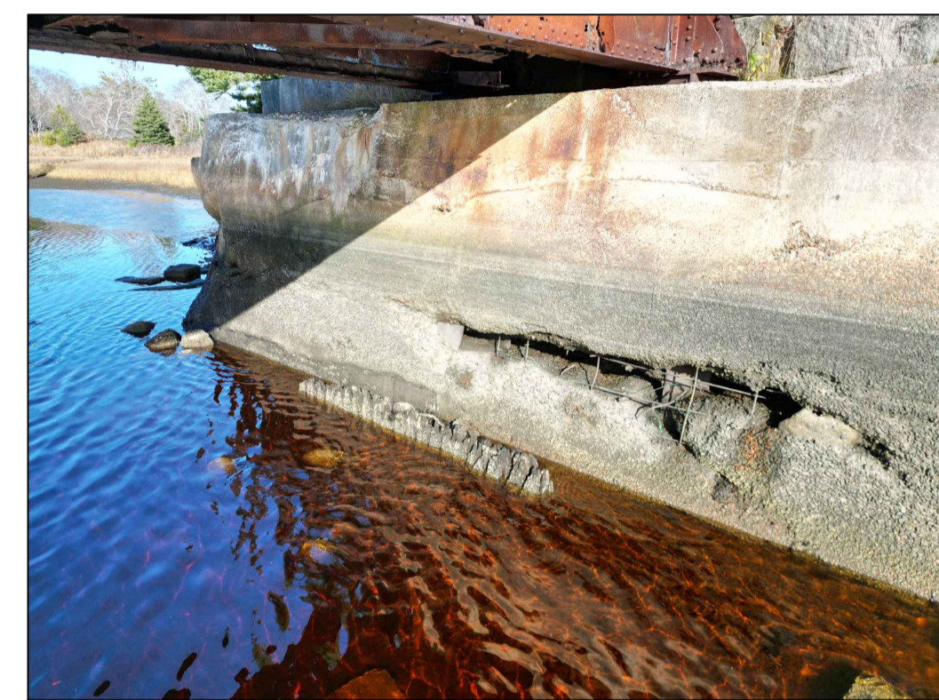
EAST ABUTMENT (CONCRETE JACKET)
