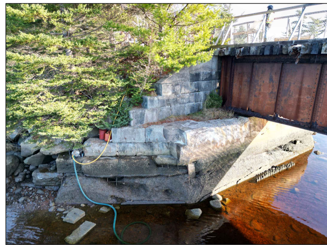
EAST ABUTMENT (OVERALL)
