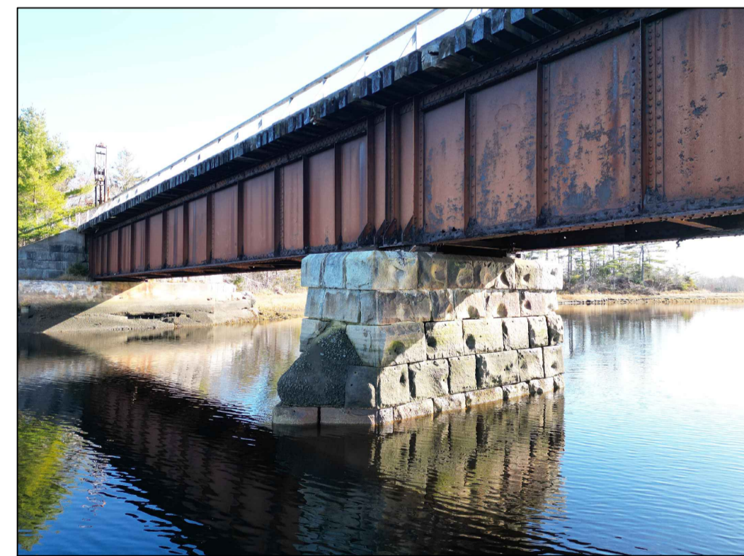
EAST PIER (OVERALL)
