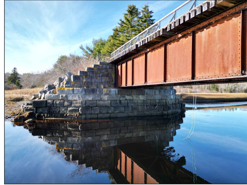
WEST ABUTMENT (OVERALL)
