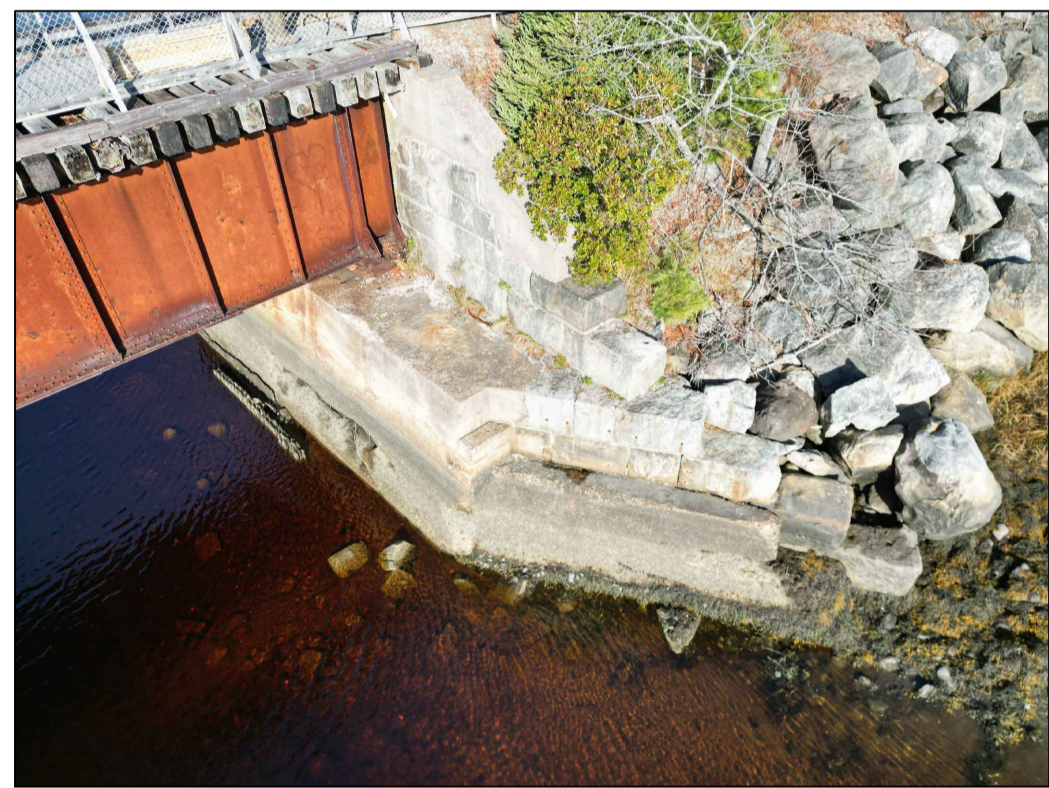
EAST ABUTMENT (SOUTH SIDE)
