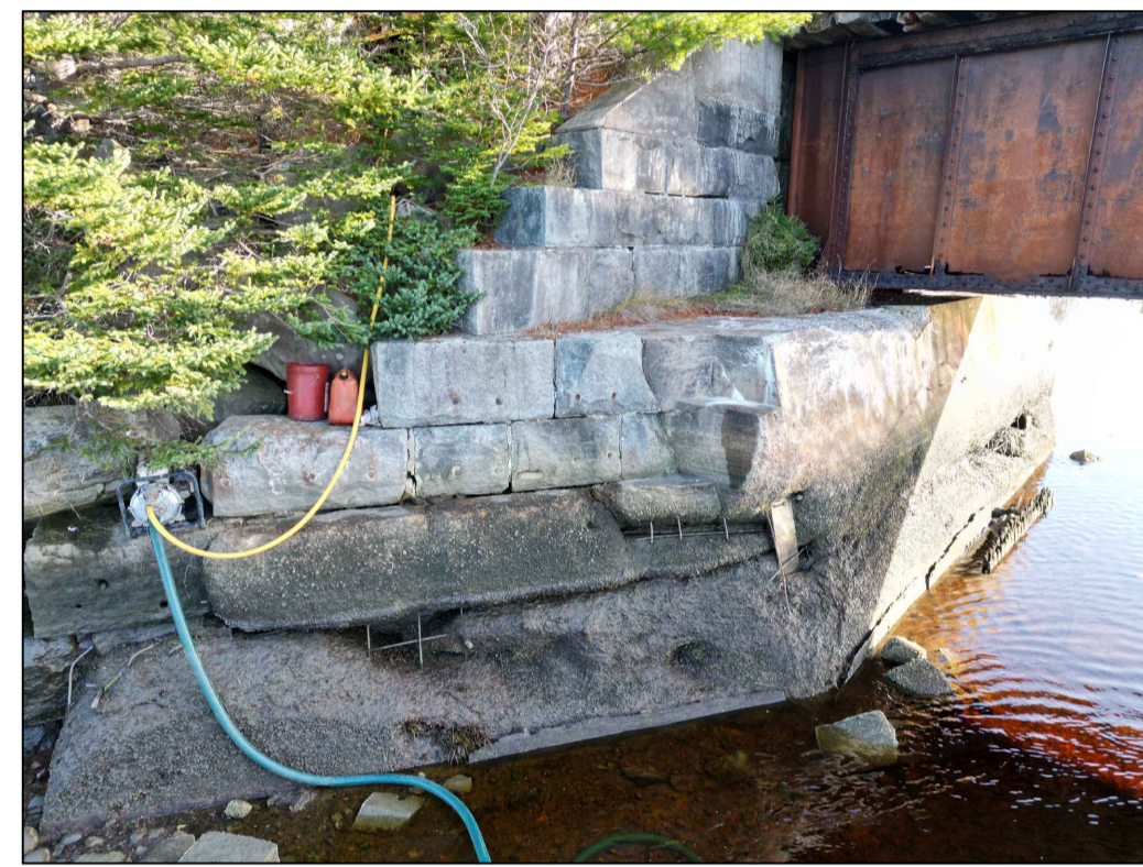
EAST ABUTMENT (NORTH SIDE)
