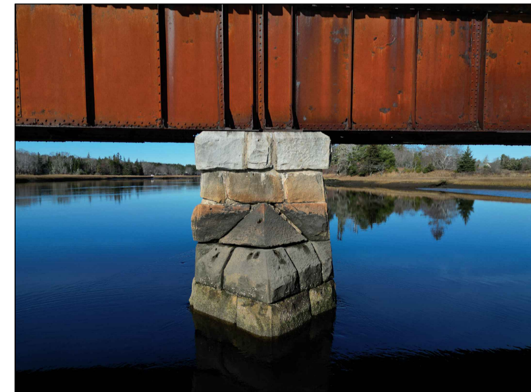
EAST PIER (NOSING)
