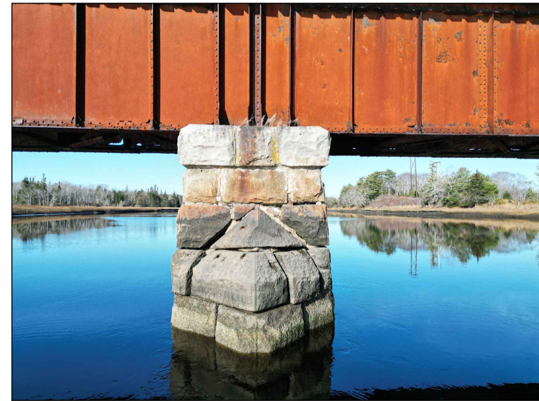
WEST PIER (NOSING)
