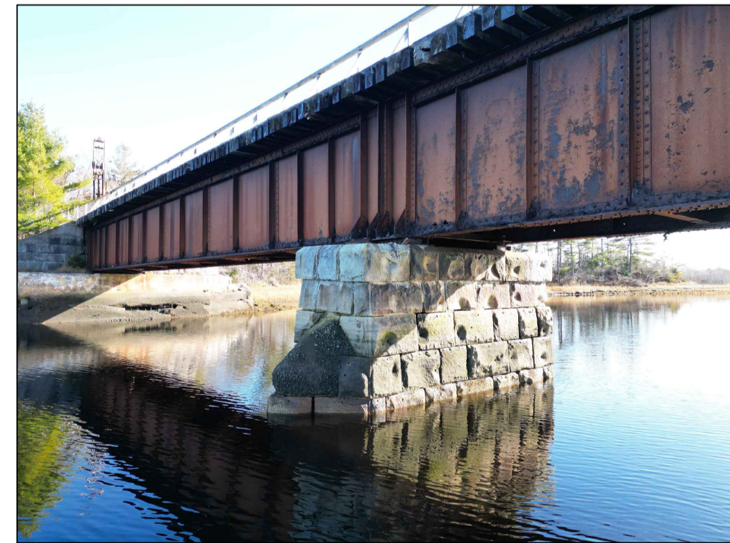
EAST PIER (OVERALL)
