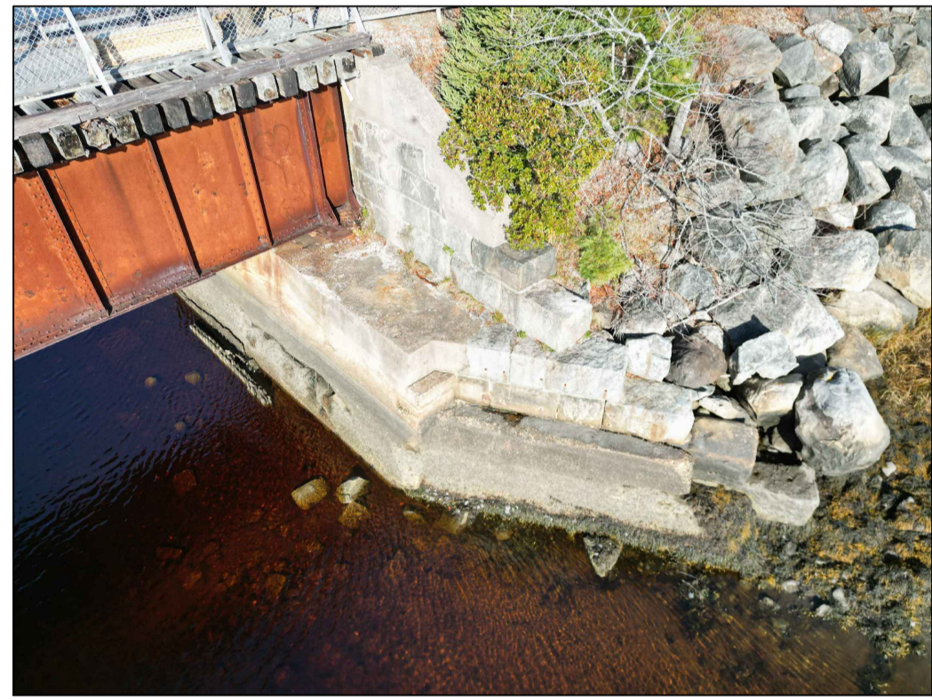
EAST ABUTMENT (SOUTH SIDE)
