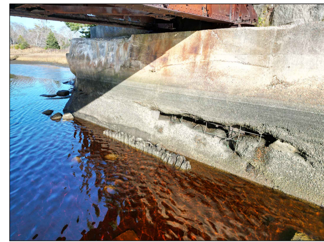
EAST ABUTMENT (CONCRETE JACKET)
