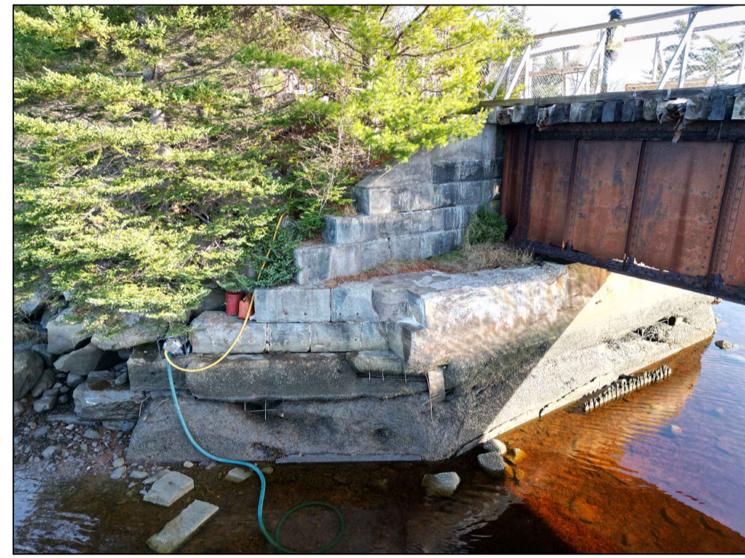
EAST ABUTMENT (OVERALL)
