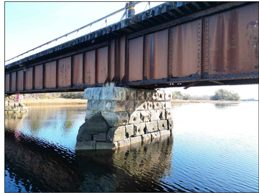
WEST PIER (OVERALL)
