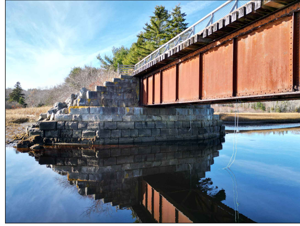
WEST ABUTMENT (OVERALL)
