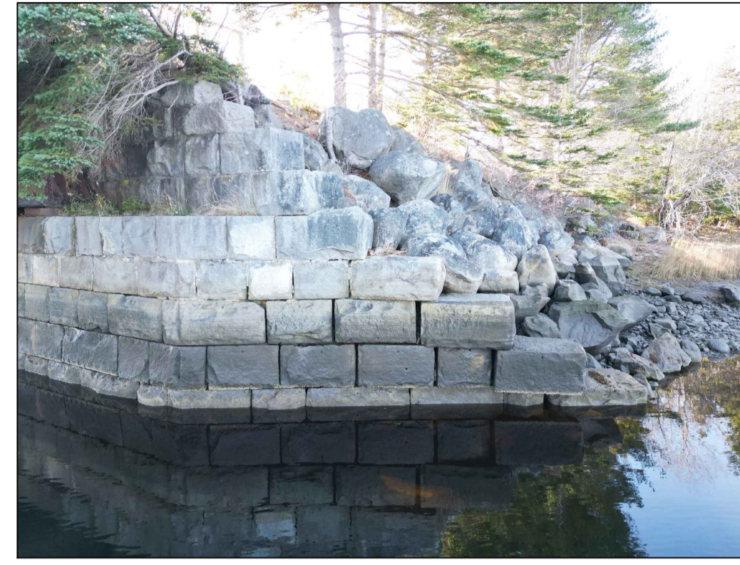
WEST ABUTMENT (NORTH SIDE)
