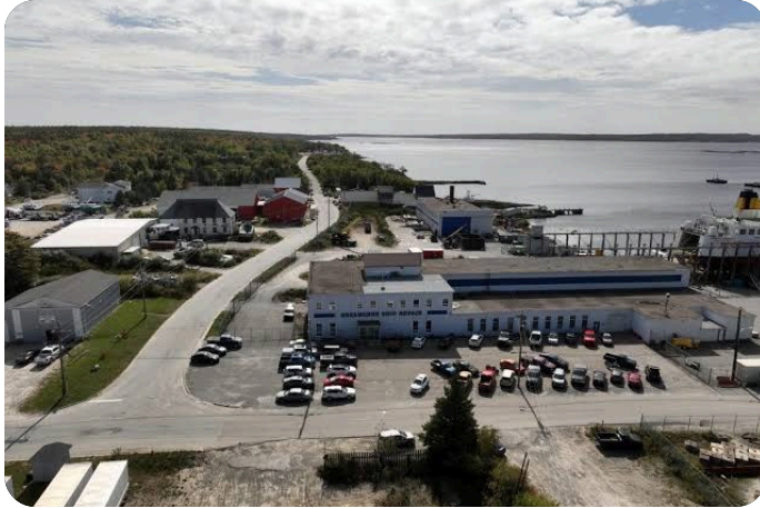
Marine industrial infrastructure on Shelburne Harbour
