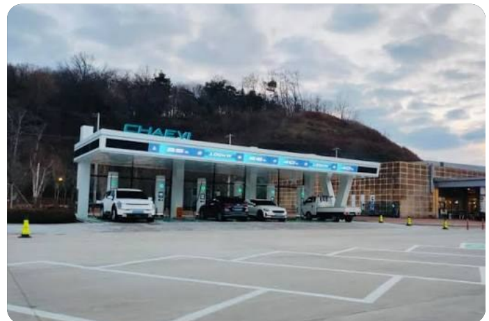
Example of the format: a canopy-covered EV charging station
