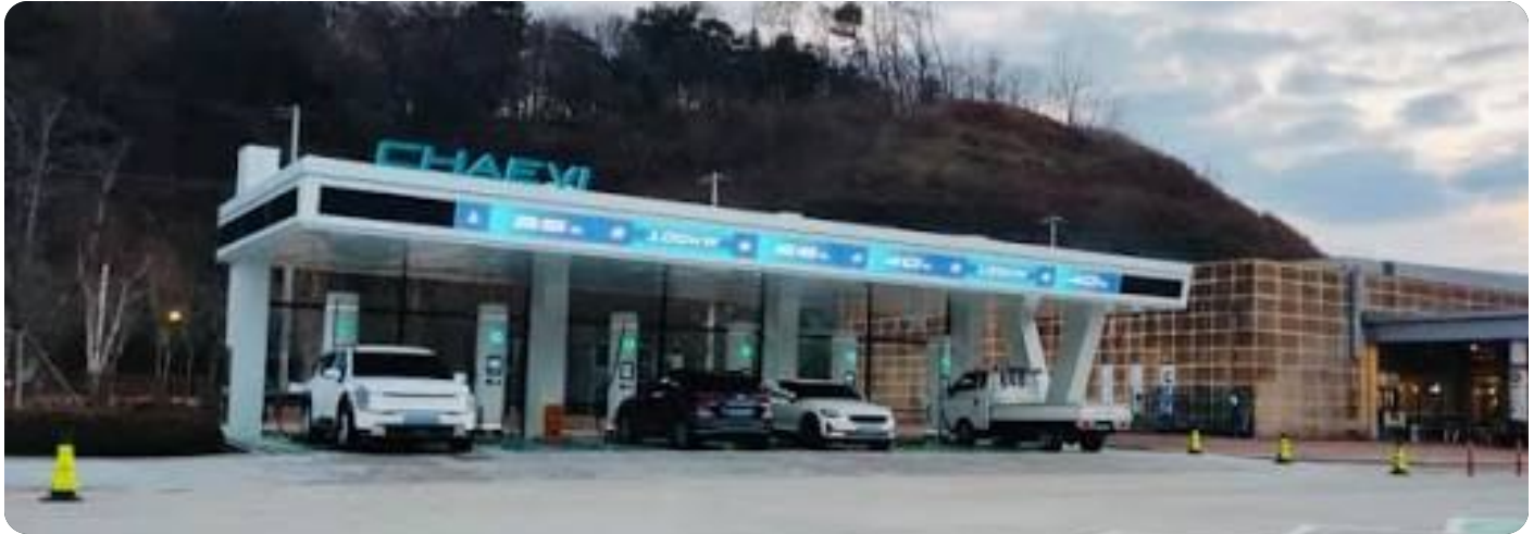
Example of the format: a canopy-covered EV charging station
