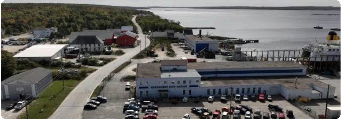
Marine industrial infrastructure on Shelburne Harbour
