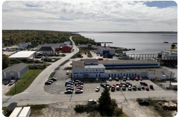
Marine industrial infrastructure on Shelburne Harbour
