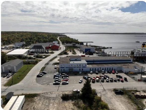
Marine industrial infrastructure on Shelburne Harbour
